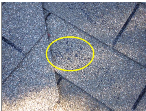
C. Photo 11 Close up view (ridge)
