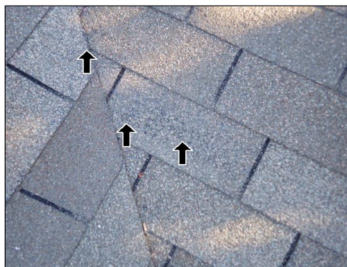
C. Photo 13 Close up view (ridge)
