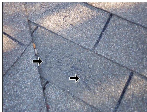
C. Photo 12 Close up view (ridge)
