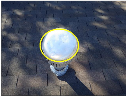
C. Photo 7 Dented spark arrester
